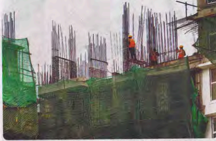
An under-construction site in Wadala where water supply has been stopped. PIC/ATUL KAMBLE
